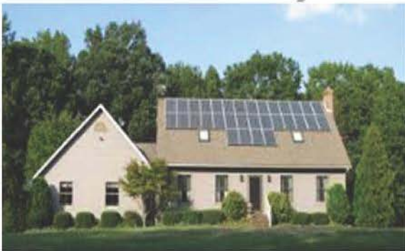
Fig. 4.8 Making use of solar energy - solar panels on a roof
