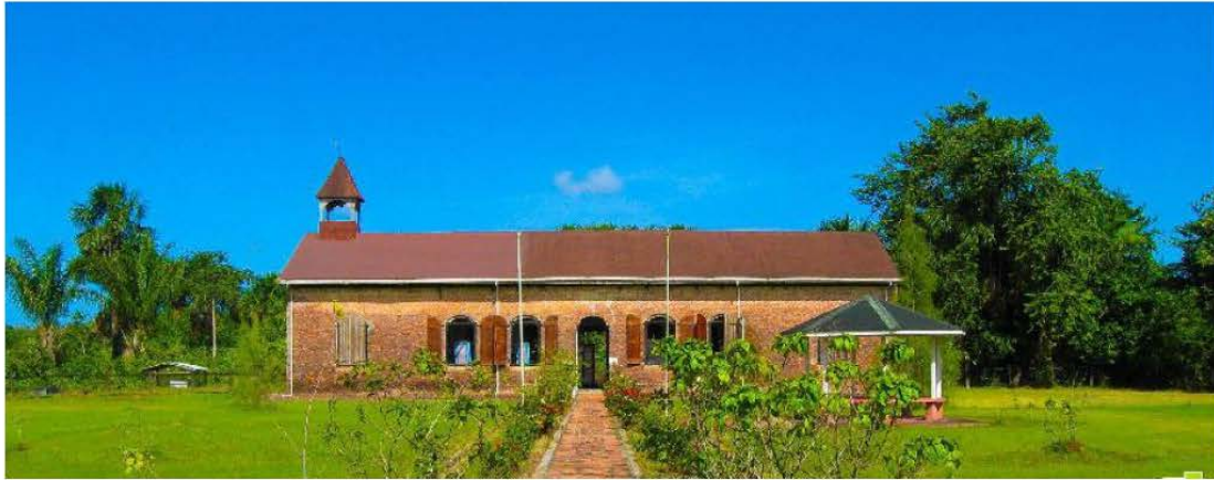
The church on Fort Island
