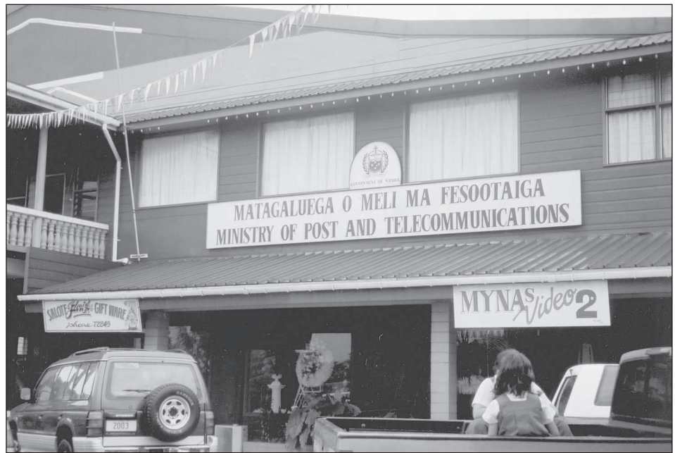
Figure 3.1H Ministry of Post and Telecommunications, Savalalo.
