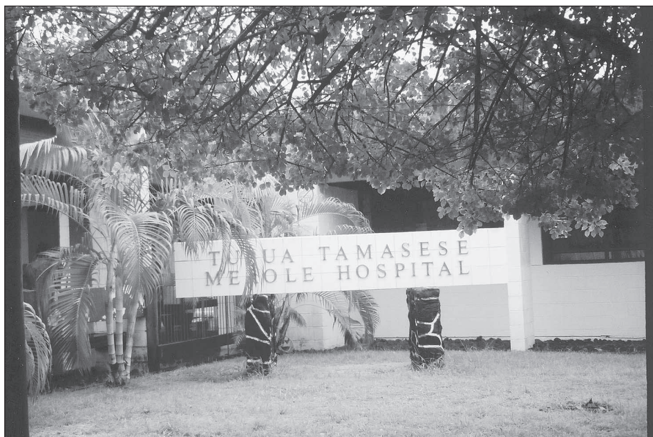
Figure 3.1E National Hospital, Moto'otua.
