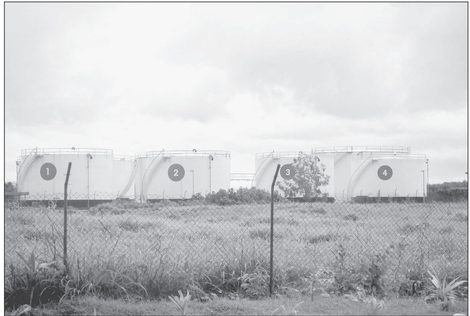
Figure 3.1G Mobil Petrol Storage Tanks, Maulinu'u.
