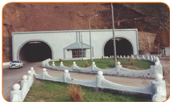
74-rasm. Qamchiq dovonidagi tunnel.
