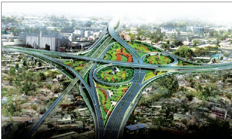
Figure 3.11 Addis Ababa Gotera Interchange Ring Road
